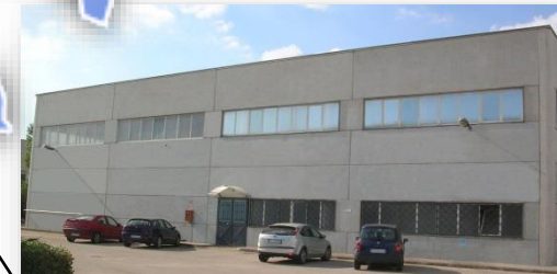
Advanced Composites Plant in ACERRA (NA)
